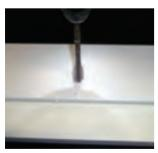
On the inside (exposed surface) of the jambs drill a 3/8" diameter hole only through the first wall no more than 1/4" deep using the 1/8" diameter holes from Step 1 as a centre guide.
